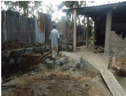
construction of a concrete fence
