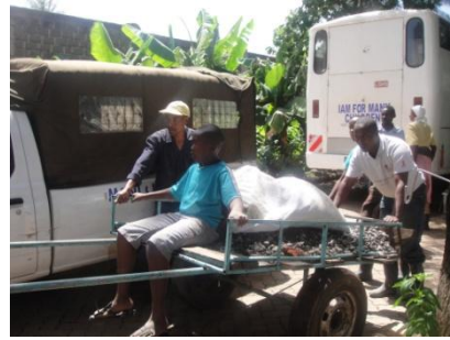
Boys transporting ballast for construction
