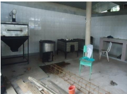
Kitchen under renovation
