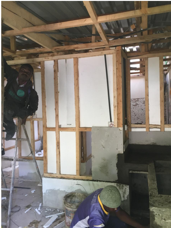
Figure 5 ongoing construction of housing unit at Imani B
