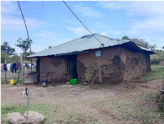
House Before Improvement
