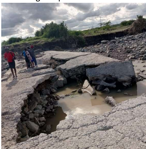
A section of the access bridge washed away by floods in 2024
