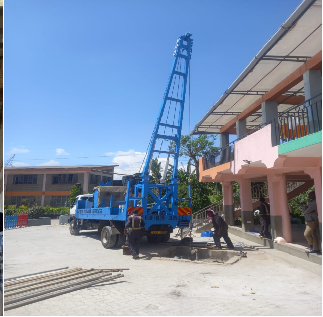
Borehole repair
