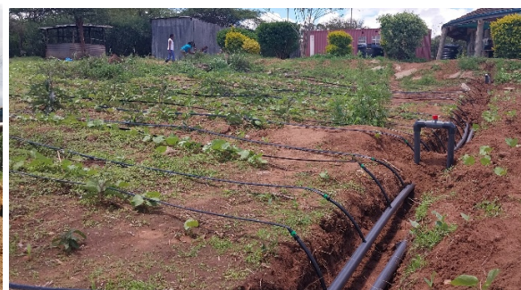
Laying of Main supply Pipes
