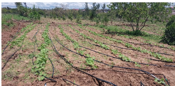
Drip line system installations
